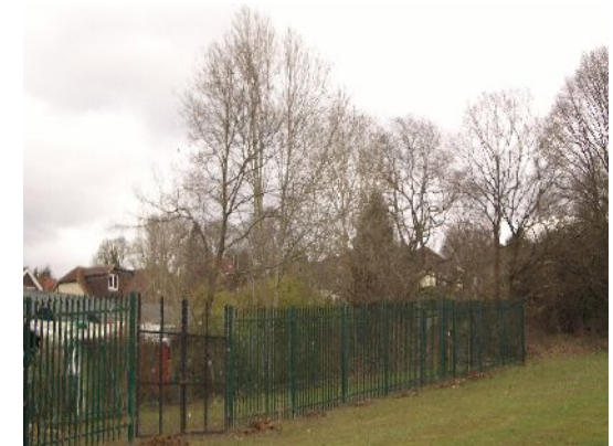
Above is the fence extension in progress and in place
